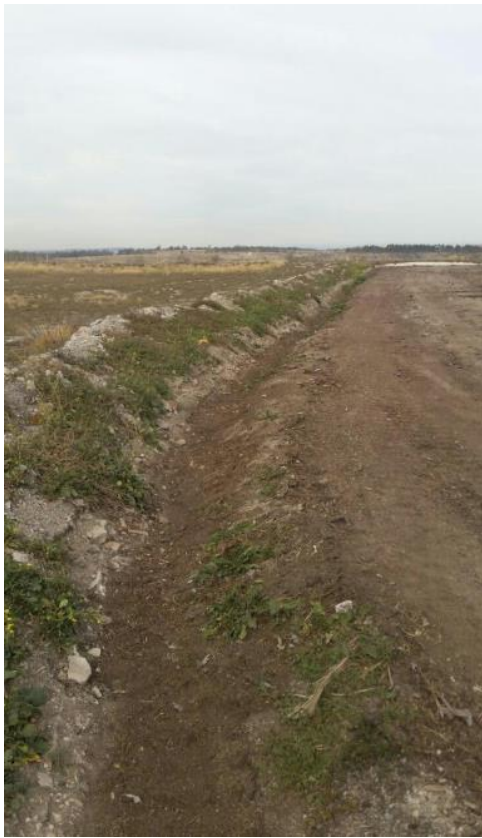
FIGURE 9: DEPICTING MOST EASTERN POINT OF NORTHERN PERIMETER DRAIN
