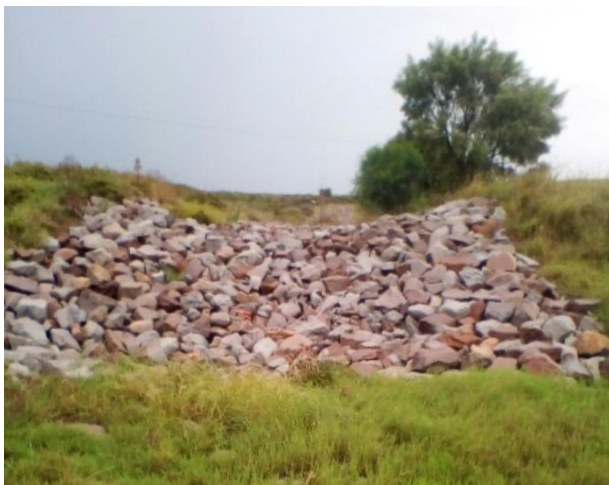
FIGURE 4: DEPICTING ENTRANCE SPILLWAY TO LOWER BASIN
