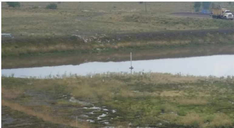
FIGURE 1: DEPICTING WATER LEVEL MARKER IN DETENTION BASIN
