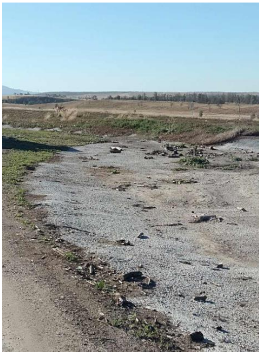
FIGURE 11: DEPICTING SHOT CRETE LINED DRAIN UPSTREAM OF DETENTION BASIN INLET SPILLWAY
